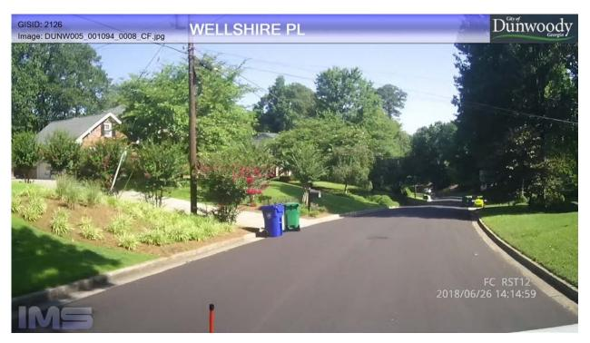
**Wellshire Place from Mount Vernon Road to Wellshire Lane (GISID 2126, PCI = 95)** – Rated as Excellent, displaying little to no surface distresses. The ride is smooth and the surface is non-weathered and the base is strong. In a couple of years, this street segment would be an ideal candidate for routine maintenance activities such as crack sealant rehabilitation.
