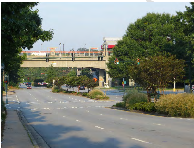
FIGURE 3. VIEW OF DUNWOODY MARTA STATION SEEN FROM HAMMOND DR
