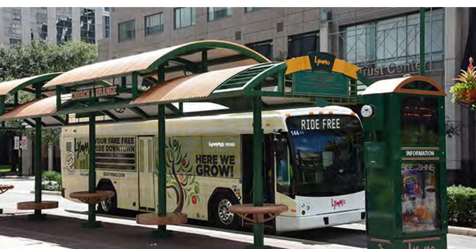
Lymmo BRT Shelter/Bus (Orlando, FL)
