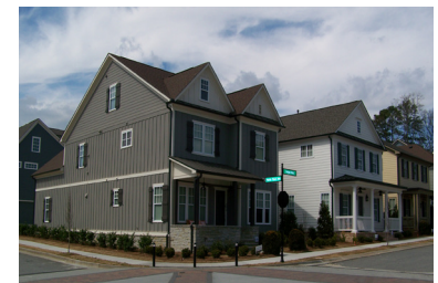
▲ New Housing in Georgetown
