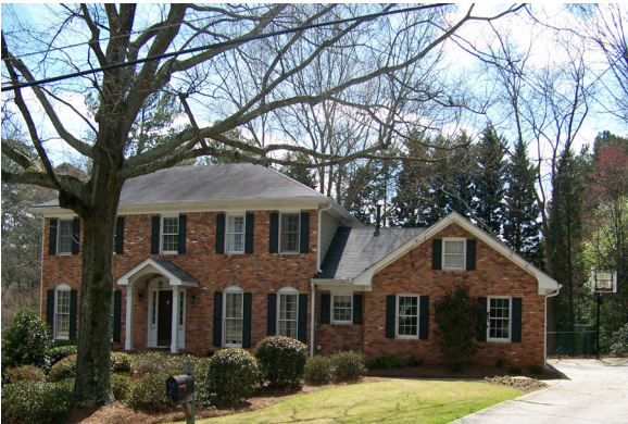
▲ Single Family Neighborhood in Dunwoody
