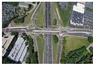
▲ Ashford Dunwoody/I-285 Interchange
