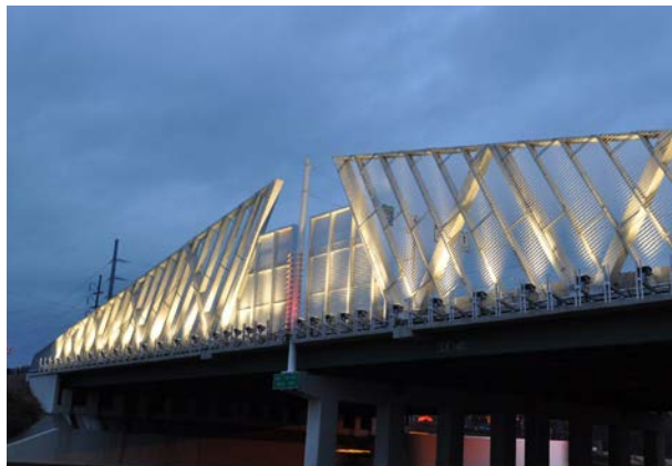
Jimmy Carter Boulevard Bridge Courtesy Gateway85 CID
