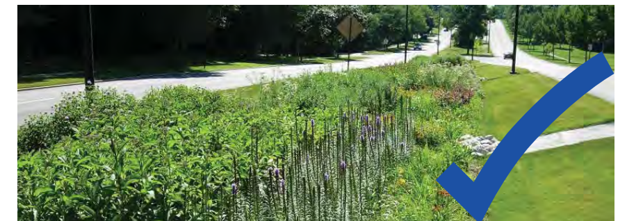
2. Bioretention Area Between Roadways
