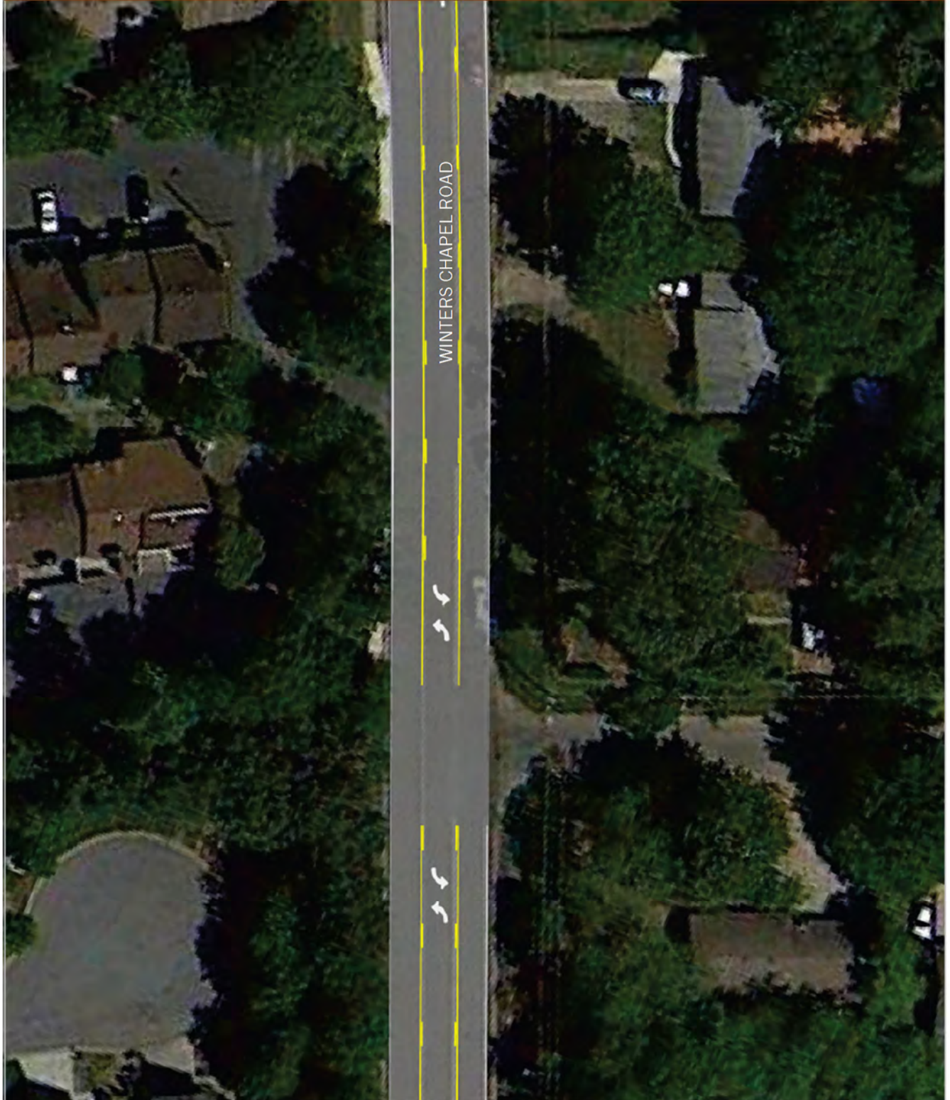
FIGURE 8 ST-5 & MT-2: USE RE-STRIPING AND WIDENING TO CREATE A CONSISTENT TWO-WAY LEFT TURN LANE BETWEEN PEELER ROAD AND SPRING DRIVE
