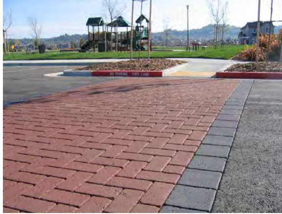
Stamped asphalt crosswalk
