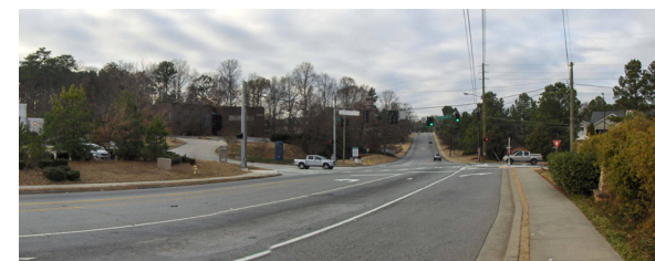
Existing North Shallowford Road at Peachford Road
