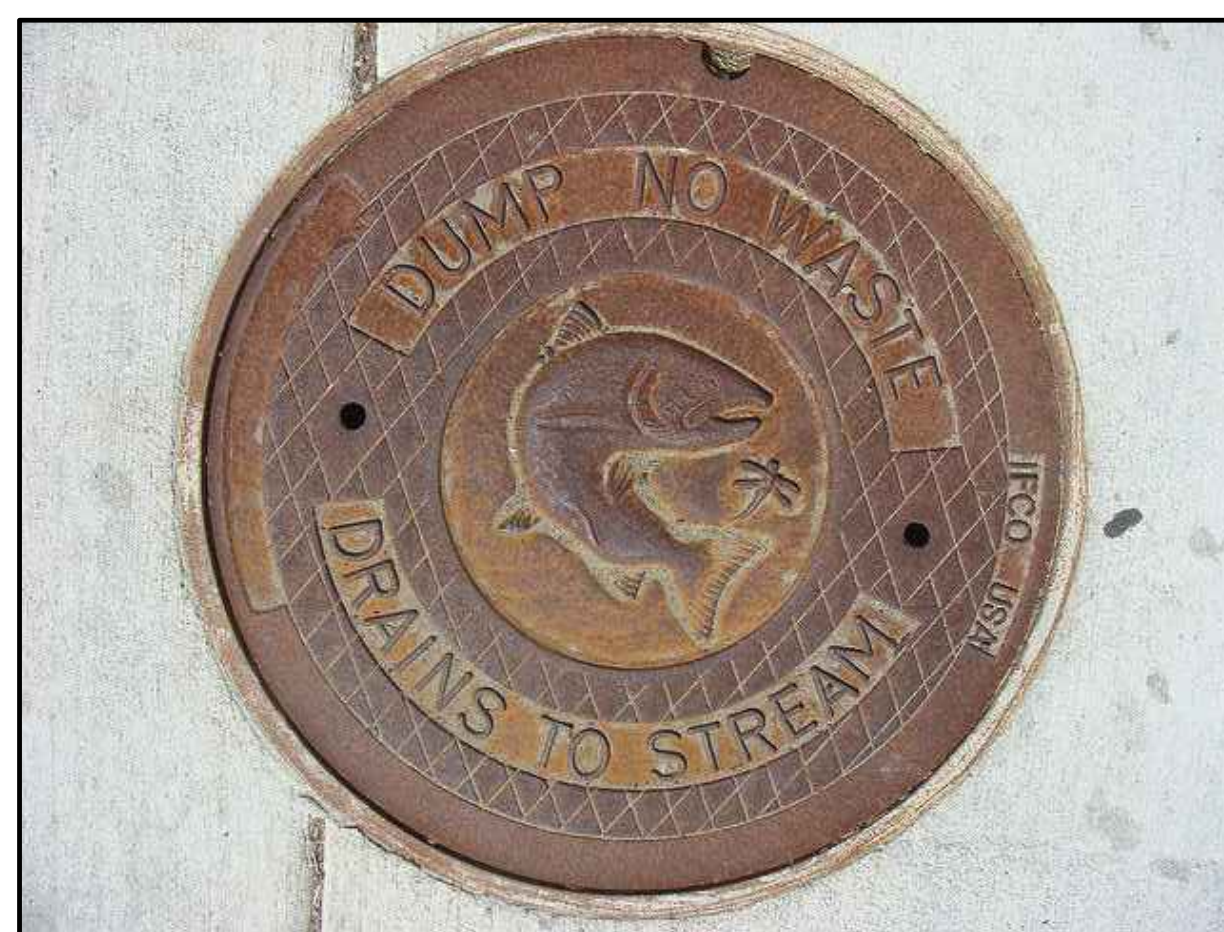
5 STORM DRAIN COVER C2.4
