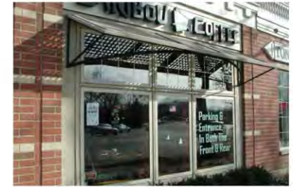
Permitted Awnings: Metal
