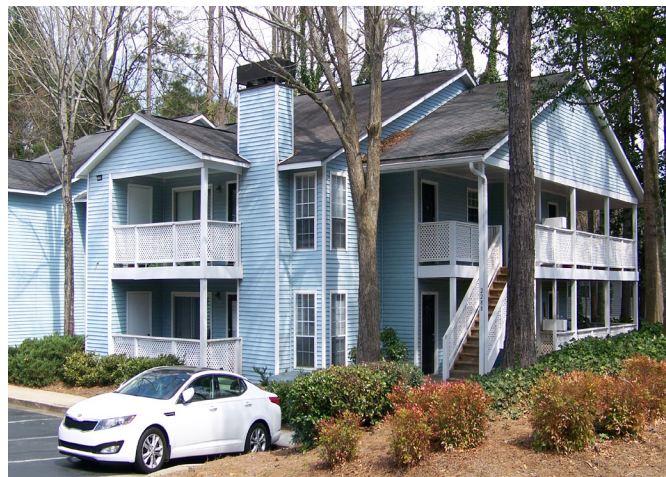
▲ Apartments off of North Peachtree Road
